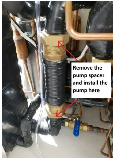
Removing the shipping spacer
